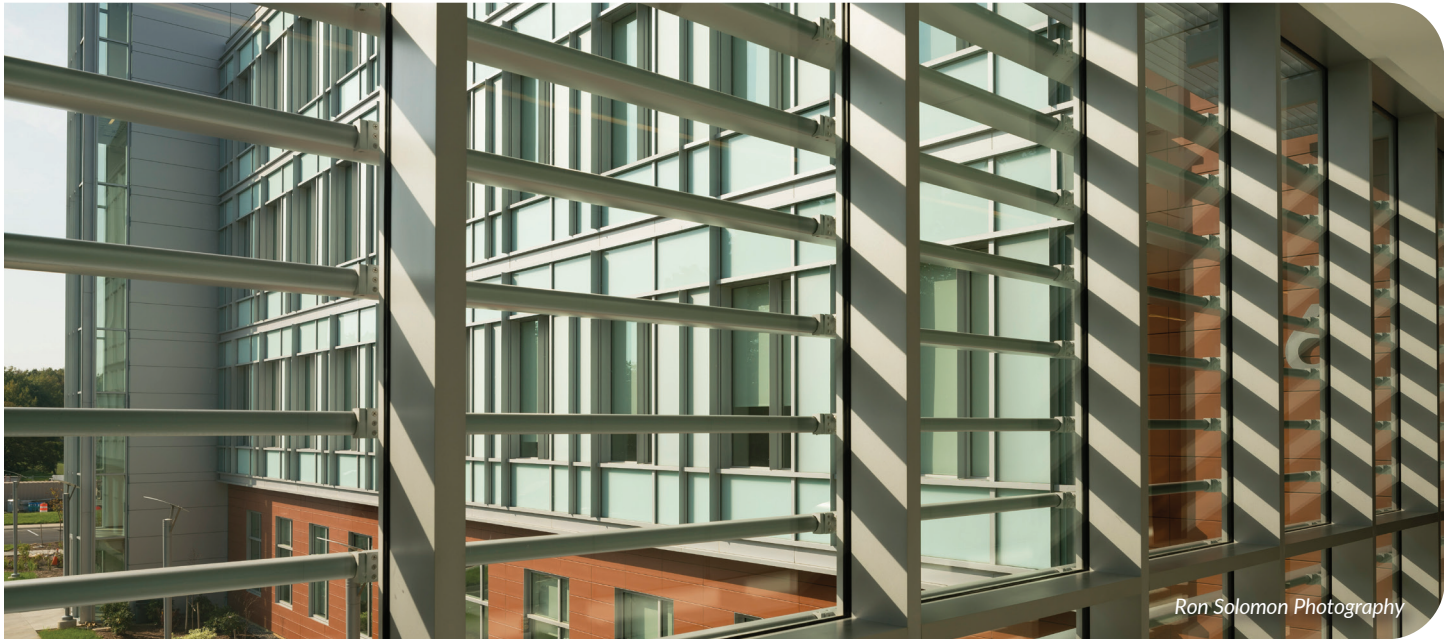
Clear, etched and spandrel glazing provides maximum daylighting, clear exterior views, outstanding glare control and high envelope insulating value at the NASA Goddard Space Flight Center, which achieved LEED® certification at the Gold level.
